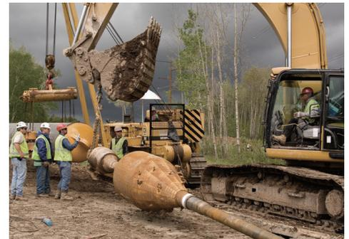
For large rivers or certain sensitive crossings, directional drilling is an appropriate and preferred construction method, depending on geologic conditions and other factors. HDD construction is considered suitable for large river crossings, extreme congestion (e.g. crossing rail yards), or other unique site-specific situations because it minimizes impacts on the area above the drill.
